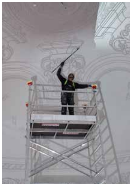
Yariv under the dome high above.
